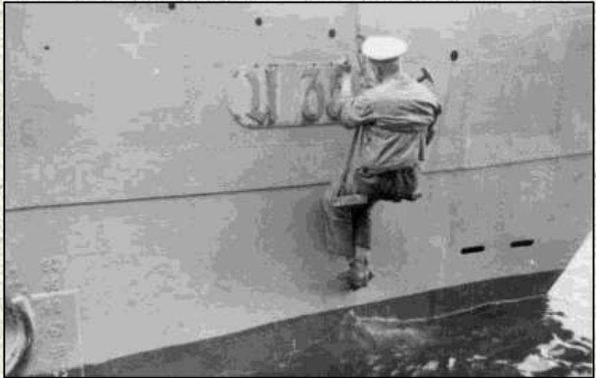
Above (33): In mid August 1939, a crewman removes a pre-war identification bow plate from the VIIA U 35 in readiness for the commencement of hostilities. At the bottom left can be seen the two-digit welded numbers, directly in front of the anchor recess, without white paint. Welded numbers have also been seen on U 30 and U 31 so it is likely that all ten VIIAs had this feature.
