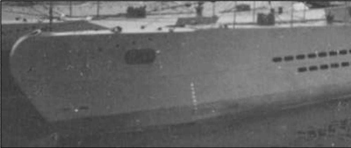
Above (7): Another image taken in the pre-war period, this time of the original VII (VIIA) U 35. The white numbers are clearly shown against the medium grey upper hull paint. Some of the numbers are not so clear against the dark grey lower hull paint. The numbers would have been present but may be obscured beneath a scumline or any slime that tended to accumulate just below the waterline of boats sitting in harbour. On VIAs, the numbers on the bow ran down to the top of the lower torpedo door.
