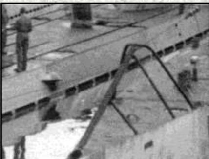
Left (58): The shroud which is part of IX outlet style 6 can be seen on the IXB U 106. There may have been slight differences in the shape of the shroud between boats and there is no painting in black around outlet style 6.
