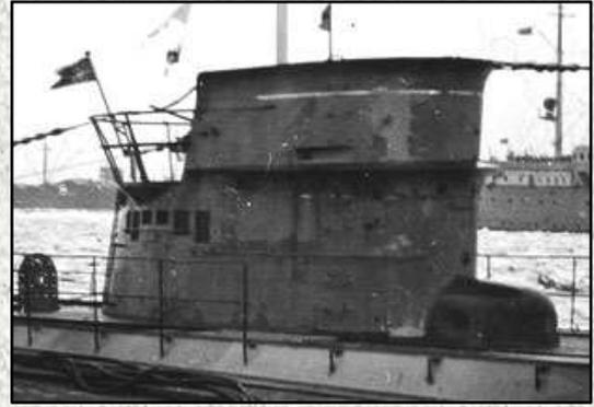
Above (2): A full length spray deflector is in place on this wartime IXA but the top of the tower still does not yet have a wind deflector.
