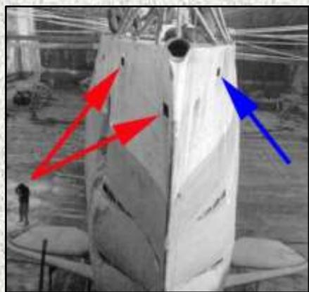
Above (65): On the IXB U 103 the two vents on the starboard side can be compared to the single vent on the port side.
