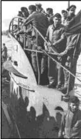
Left (D12): The very low height of the tower can be seen in this photo in which the top of the bulwark only comes up to chest height. It is easy to appreciate why the curved railing bars needed to be added above the tower.
