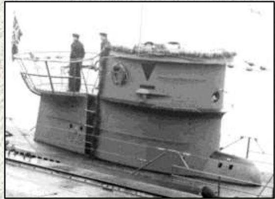
Above (6): The standard magnetic compass fairing on U 408. As the photo illustrates, the fairing abutted the front of the tower.
